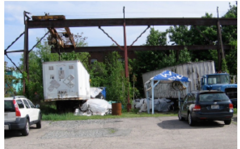
view of gantry above trailers
